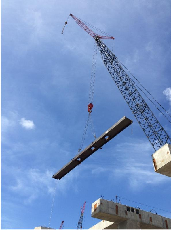
The ring beam is a major component of the train structure and is comprised of large, angled columns that are joined in a ring at the top by post-tensioned concrete. Some of the largest beams of steel will be bolted to other beams to create spans more than 70 feet long that will support the widest parts of the ring beam.
