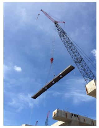
The ring beam is a major component of the train structure and is comprised of large, angled columns that are joined in a ring at the top by post- tensioned concrete. Some of the largest beams of steel will be bolted to other beams to create spans more than 70 feet long that will support the widest parts of the ring beam.
