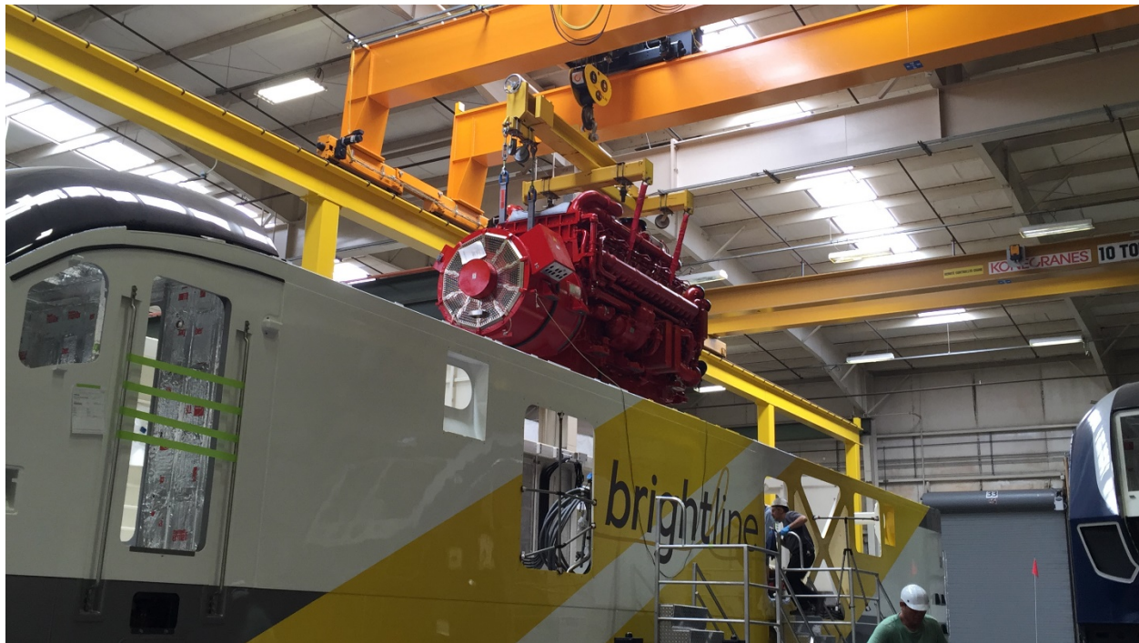
The 31,000 pound Cummins engine is lowered into the first Brightline locomotive.
